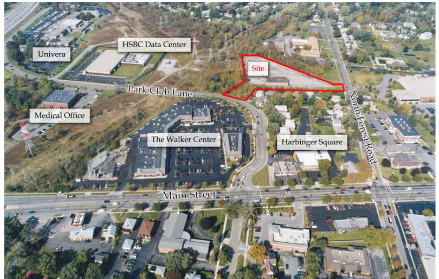
Iskalo Development acquired a former National Grid service center at 70 North Forest, Williamsville, NY, in close proximity to the intersection of North Forest and Main Street.
