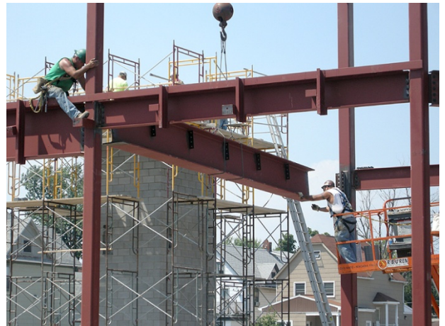
Crews will now begin work on the building's exterior shell.
